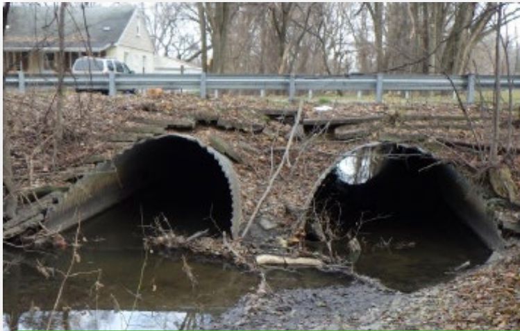
Ecorse Creek Culverts
